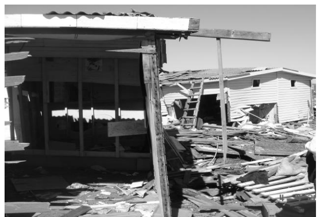
Fig. 2 Destroyed houses behind the sand dunes
