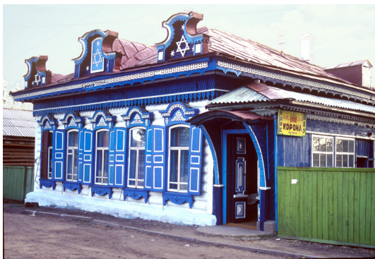
Fig. 11. Nerchinsk. Wooden house and store, Soviet Street 12. Photograph: William Brumfield (9/12/2000)
