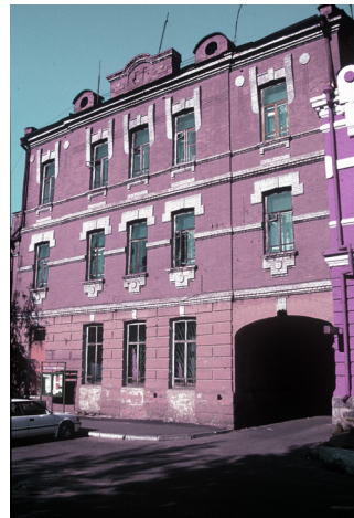
Fig. 18. Chita. A.E. Dukhoi Building, Nerchinsk Street 19. Photograph: William Brumfield (9/14/2000)
