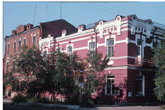
Fig. 19. Chita. A.E. Dukhoi Building, Nerchinsk Street 21. Photograph: William Brumfield (9/14/2000)
