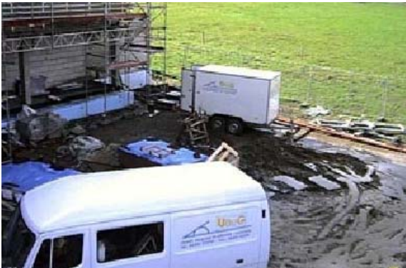
Figure 12: TRT-equipment of UBeG GbR on site for design of a BHE field in Aachen, Germany
