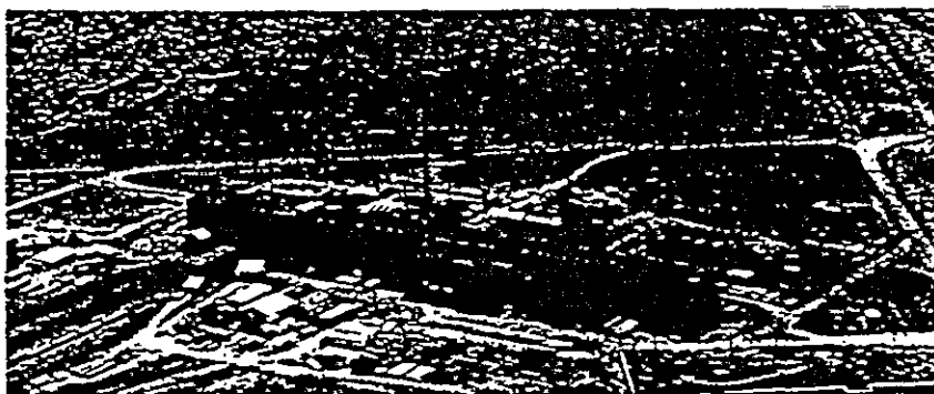
These 1994 photographs show T Plant and B Plant, two of the earliest separation facilities on the Hanford Site. These plants are about 800 feet in length and 100 feet in height (includes both above and below ground portions).
