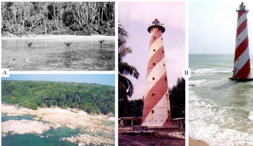
Figure 7A Historic view of North Sentinel island shoreline (courtesy George Weber) compared to an Indian Coastguard photo after the earthquake. Uplift here is estimated to be 1-2 m with the pre-earthquake coral lagoon now completely raised above mean sea level. Figure 7B are views of Indira Point lighthouse (6°45.2'N 93°49.6'E) c. 1980 compared to Indian Coastguard photo of flooded base of lighthouse after the earthquake. Subsidence here is estimated to be 4.25 m based on its foundation being 3.5 m above sea level when constructed, and in January 2005, level with low tide, and submerged 1.5 m at high tide. The steel shell lighthouses, like that at Indira Point, fared well in the earthquake, but masonry lighthouses at Interview Island and Katchall island were badly damaged.
