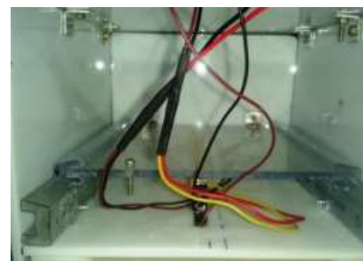
Fig 3. Internal view of the box
