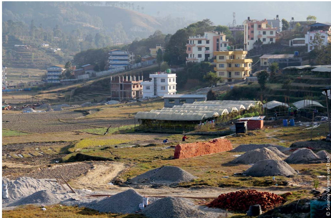
FIGURE 1: Brick-making for the vibrant construction sector is competing with efforts to intensify agriculture close to Dhulikhel, Nepal. Guiding efforts towards achieving the Sustainable Development Goals requires assessing not only benefits and trade-offs, but also assessing who gains and who loses at the local level.
