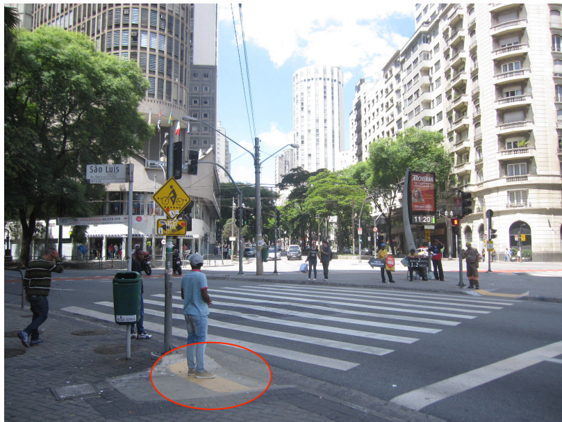
Figure 6 – Low floor without a warning/sign.
