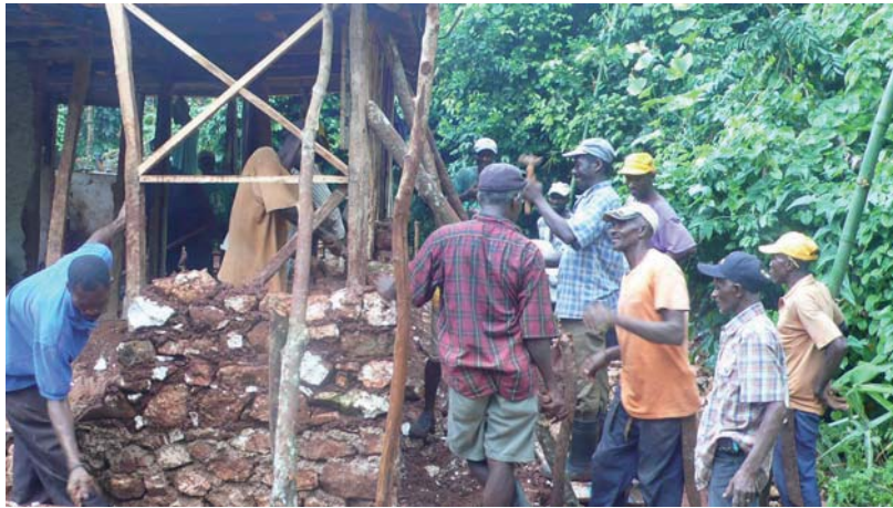
Fig.2 – Haiti, Cap Rouge: training of local masons for housing repair (credits: CRAterre, 2010).
