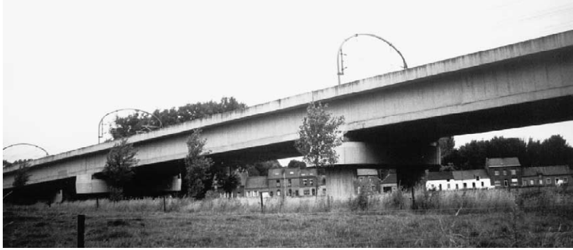
Fig. 4. View of the Antoing Bridge.
