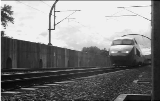
Fig. 9. Dynamic experiment of Antoing Bridge.
