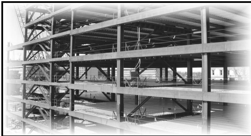
Figure 1.1: Bracing Systems
