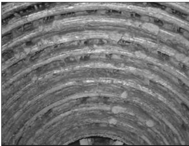
FIG. 19. Close-up of heat exchanger non-uniform deposit.
