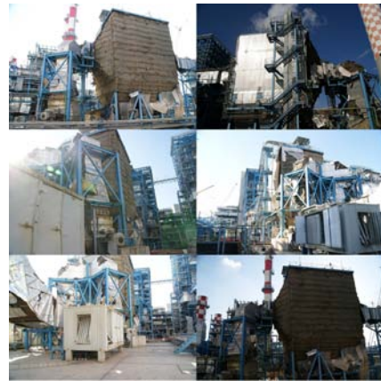
Figure 3. Different views of the Electricity station under varying illumination conditions.
