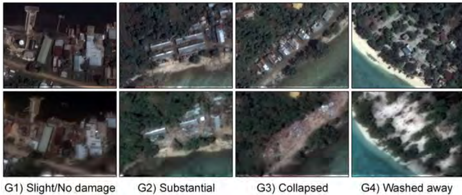
Fig. 11. The structural damage interpretation is divided into four classes: slight/no damage, substantial damage, collapsed and washed away
