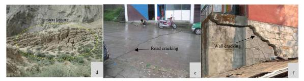
**Figure 4.** Typical landslides and their impacts on residents within the study area. (a) Lunba Landslide in a tributary. (b) Zhuolonglang landslide in Jiayu County. (c) Mentang power station landslide. (d) Landslide due to a tension fissure in Danglaimu. (e) Sino-Nepalese Highway cracking. (f) Wall cracking in a Public Security Bureau computer room.
