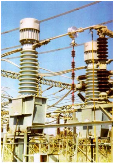
Figure 1 - FOCT with fibre optic composite high voltage downlink
