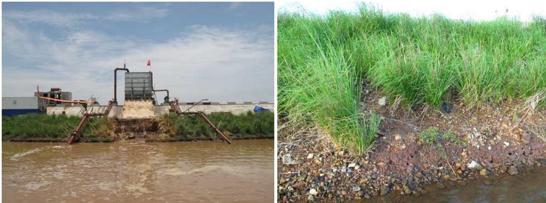
**Figure 2. Left: Simulator on dike crest in Hai Phong. Right: lower part of the landward slope was covered with vetiver grass.**
