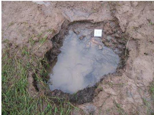
Figure 11. Damage at transition between dike slope and dike toe.
