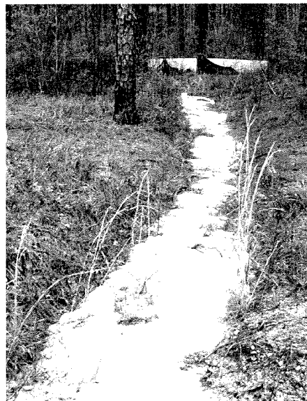
Typical sediment plume development downslope of a forest road turn-out section.
