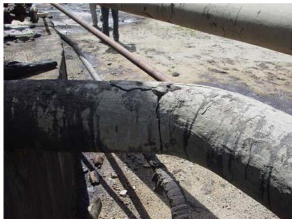
*Figure 4. Cracks observed on tank piping system*
