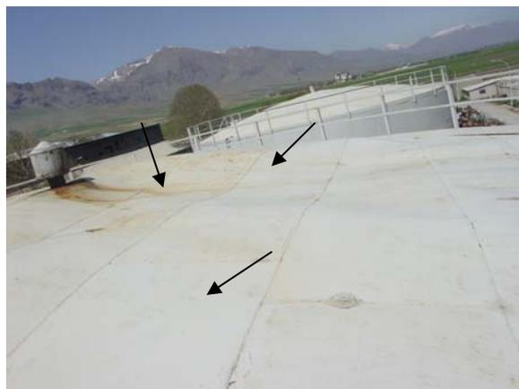
*Figure 5. Damage to tank roof*
