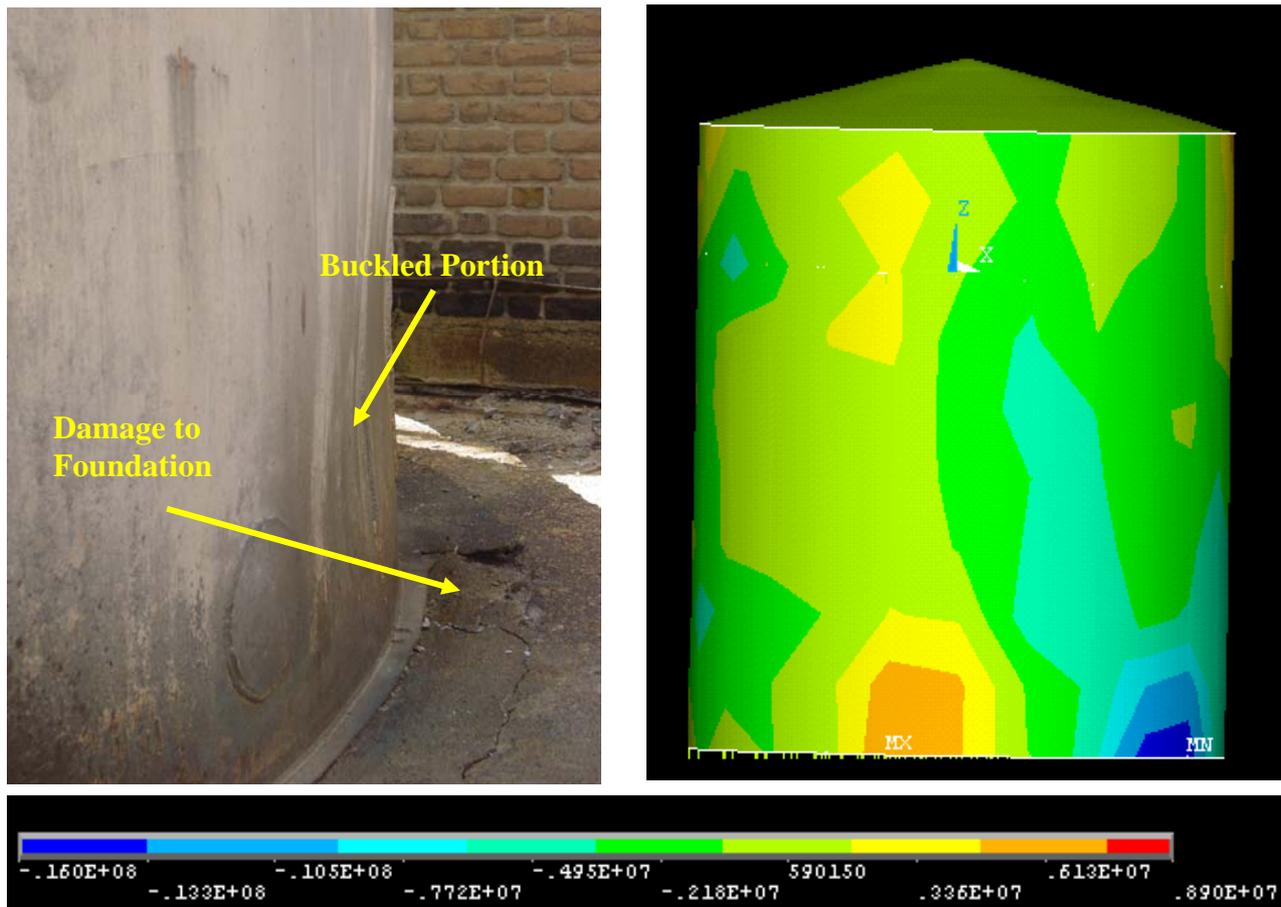
*Figure 6. Tank T2 Shell buckling; actual behaviour compared with finite element analysis.*
