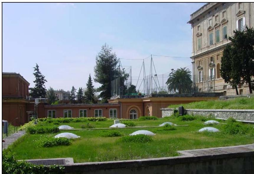
The first phase of the monitoring programme was carried out in May 2007 during the retrofitting works for the new green roof system, when the rooftop was only covered with the impermeable layer in order to measure the hydrologic response of the impervious roof. The impervious system was modelled by employing the EPA Storm Water Management Model (SWMM 5.0) to obtain a virtual reference impervious roof for comparison with the green roof hydraulic performance.
