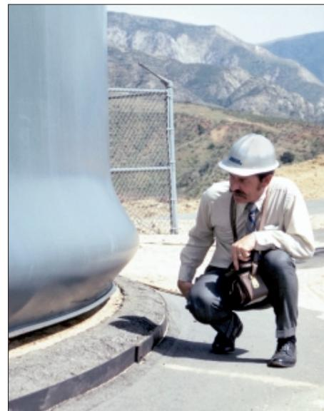
Fig. 1: Elephant-foot buckling of a tank wall (courtesy of University of California at Berkeley)
