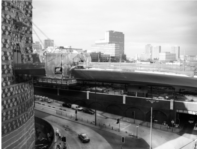
Figure 01. The bridge in on site March 2003, without canopy.
