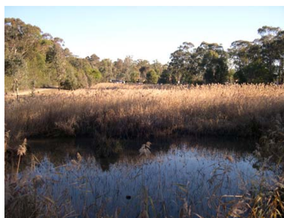
Figure 1. Free water surface constructed wetland for stormwater runoff treatment in Plumpton Park, NWS, Australia. Photo author.
