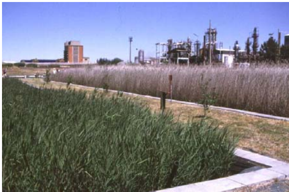
Figure 6. HF constructed wetland at Estarreja, Portugal treating wastewaters from nitric acid production. Photo author.
