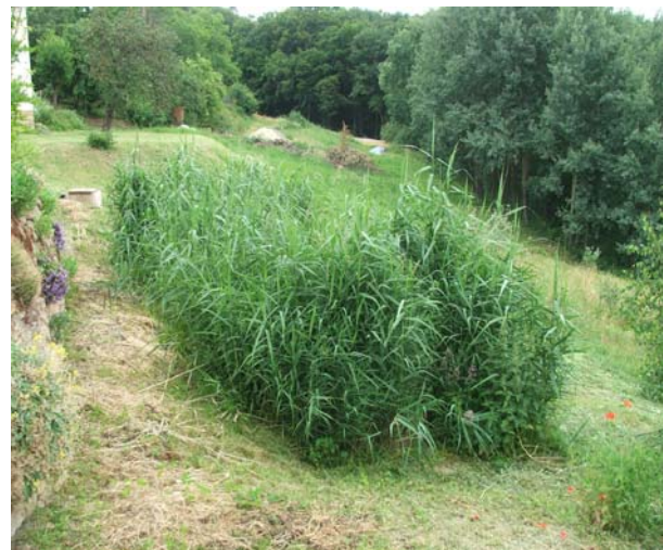
Figure 4. HF constructed wetland for 5 PE in Kostelec nad Černými Lesy, Czech Republic planted with Phragmites australis . Photo author.
