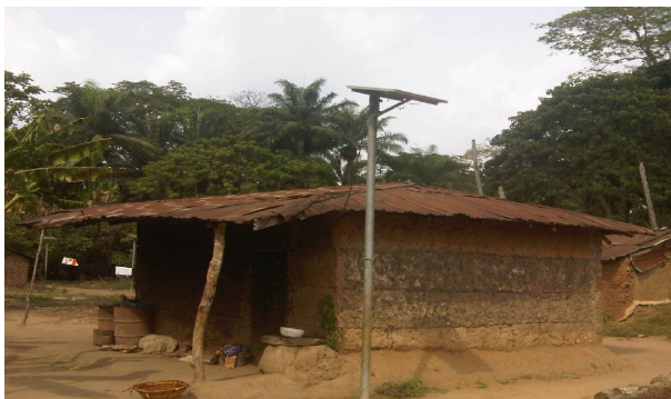
Figure 3. Installed home solar lights.
