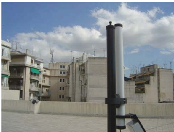
Fig. 13 – PMM8057 station at Kipseli, Athens.
