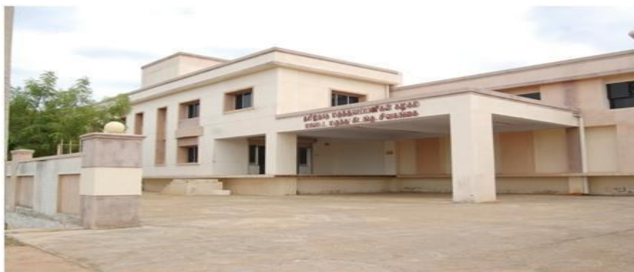
Fig. 4: TNMSC Warehouse at Sivagangai
