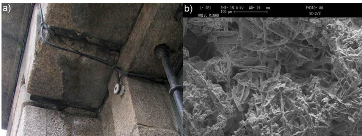
**Figure 5.** Example of carbonate crusts on granite stones.
