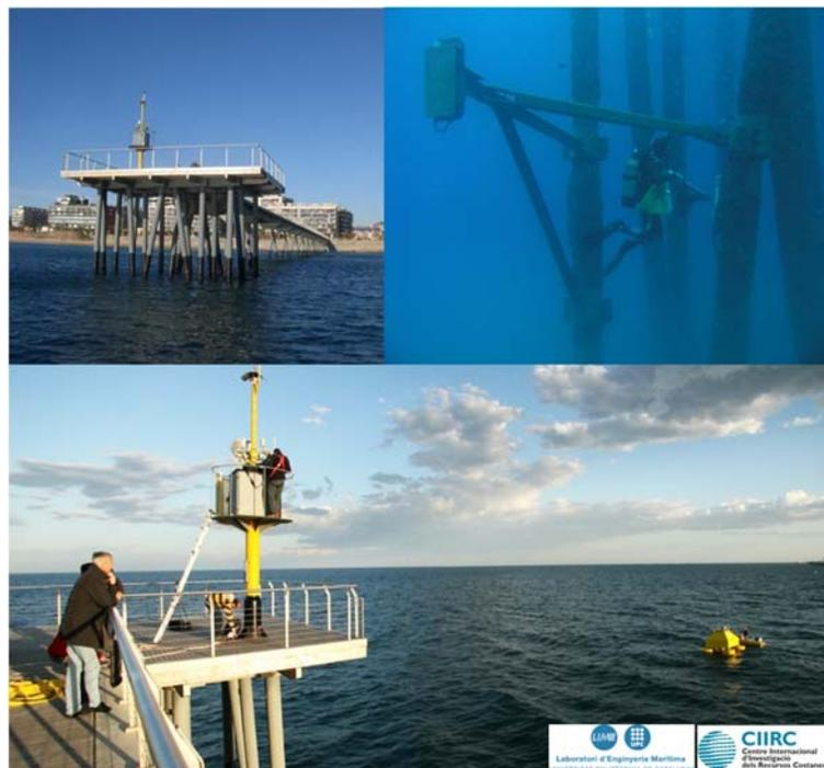
**Figure 4. Sample illustrations of the instrumented coastal pier scientifically managed by UPC in Barcelona and located off the Badalona coast. The upper left panel shows an overall picture of the pier type (at a water depth of about 13m) while the upper right and lower panel illustrate the deployment of observational equipment in one of the legs and for the testing of a floating buoy.**
