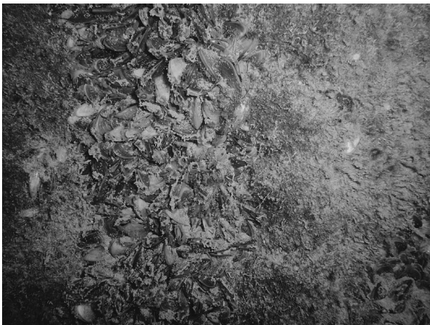
Fig. 3. Photograph of golden mussels attached to an artificial concrete bank of the Tone River.
