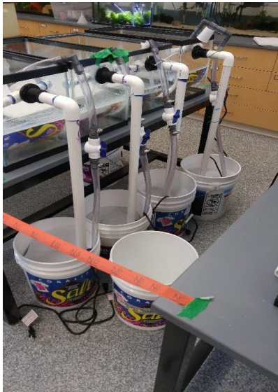
Figure 1. Portrays the plumbing system that goes from the tank to the buckets below.
