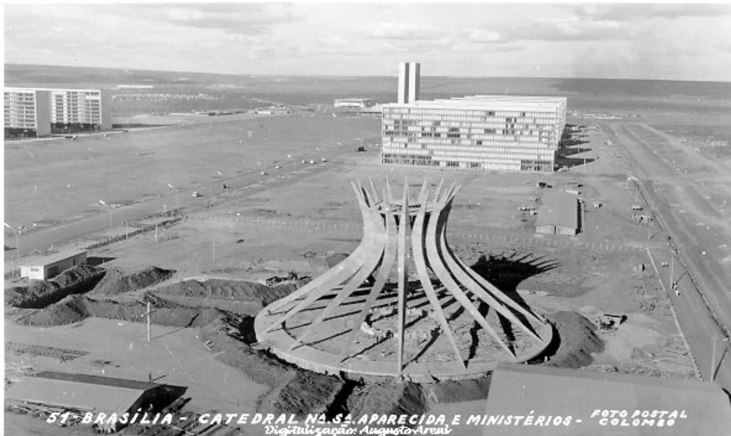
Fig. 2 Brasília Cathedral, with the structure just poured, before the inauguration of Brasília (unknown photographer).
