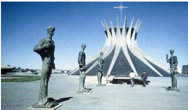
Fig. 3 Brasília Cathedral, with exposed concrete structure and lateral sheathing between the piers (photo: Alexander Fils).
