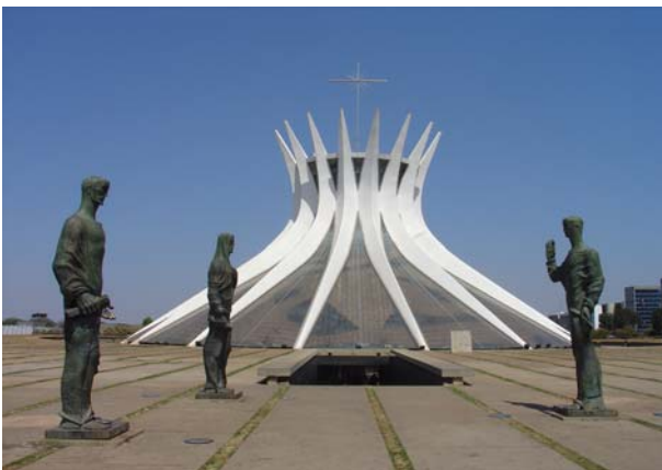
Fig. 4 Brasilia Cathedral, present state: view towards the outer access ramp.
