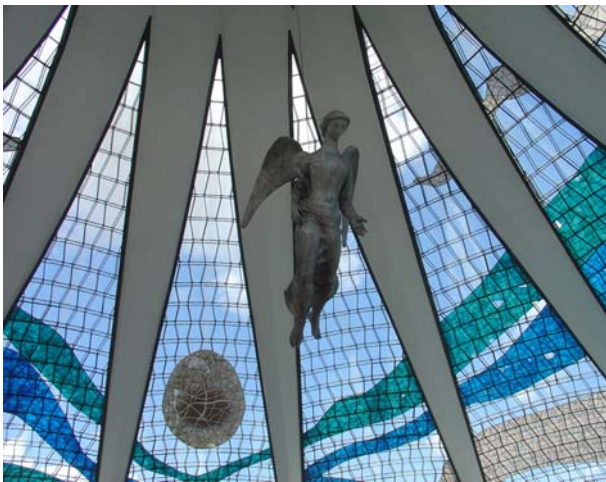
Fig. 11 The spatial frame between the piers allows the fastening of two layers of glazing on the upper and lower hexagonal webs of the truss (photo: author).
