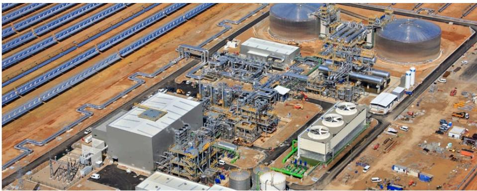
**Figure 1.** General view of “La Africana”. Hot and cold tanks are shown at the top, with the heat exchanger in between. The solar collectors are located at the left of the image.
