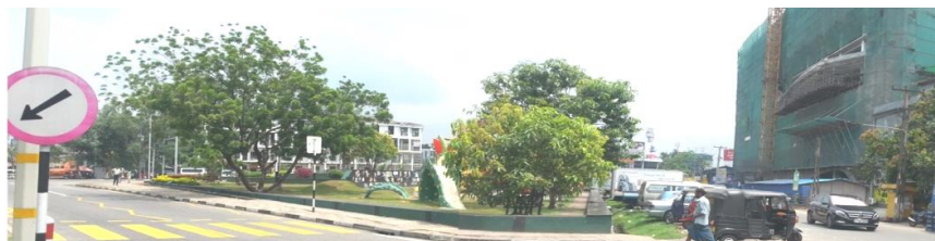
Fig 41: C-1 Rajagiriya Children's Park with surrounding pedestrian path, on street parking and elevated functional space
