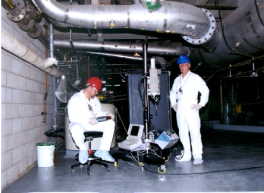
Fig. 5. A very large overhead duct is measured from below with a portable, collimated HPGe detector. The measurement distance for any detector positioned beneath this duct will be comparable to the duct diameter because of the limited height of the equipment above the floor. For common ventilation ducts such as these, the duct width is always a significant fraction of the width of the field of view of the collimated gamma-ray detector. In this case, the duct surface completely fills the field of view of the collimated detector, a geometry that should be (depending on the dimensions of the deposit) best-suited to the GGH assay of an area deposit.
