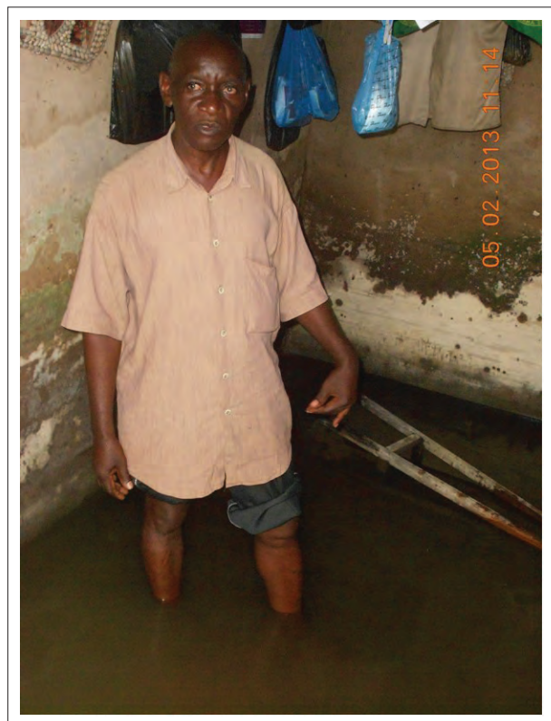
FIGURE 6: Dampness and waterlogging inside a house in Keko Machungwa resulting from underground water percolation.
