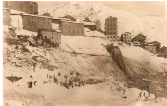
Figure 3. Damages on buildings and Rebolledo Bridge caused by the avalanche of 1941 (source: Sewell Museum).
