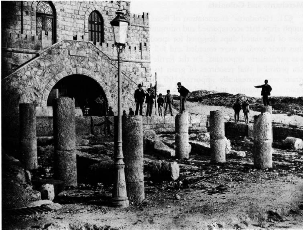
FIGURE S.4. A LATE-NINETEENTH-CENTURY PHOTOGRAPH OF THE REMAINS OF FOUNDATIONS AND COLUMN SUPPORTS OF THE ATHENIAN SHIPSHEDS AT PEIRAEIUS.
