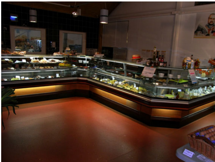
Figure 5.10 Typical serve-over refrigerated retail cabinet display.
