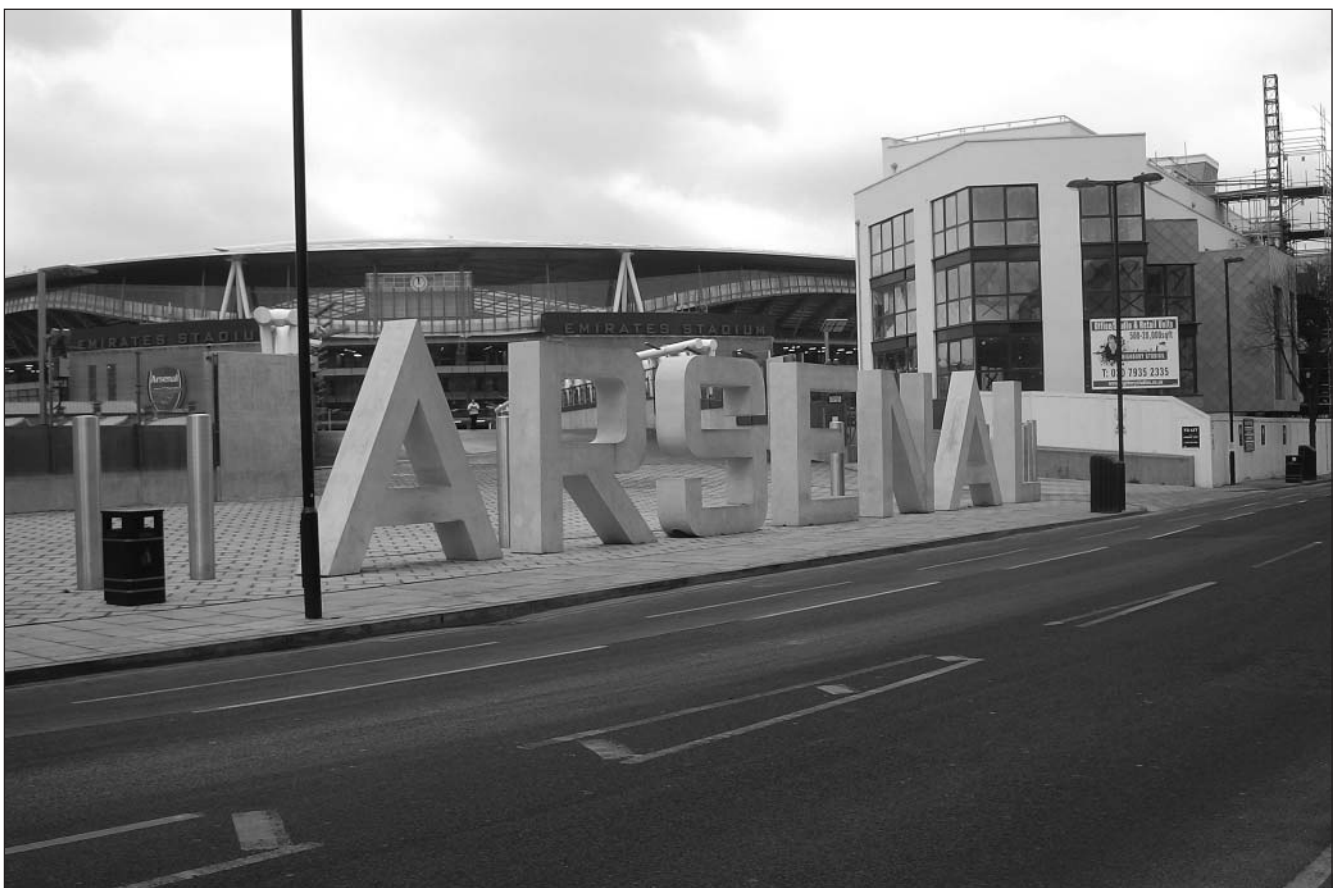
Fig. 5. The reinforced concrete barrier at an entrance to the Emirates stadium, north London
