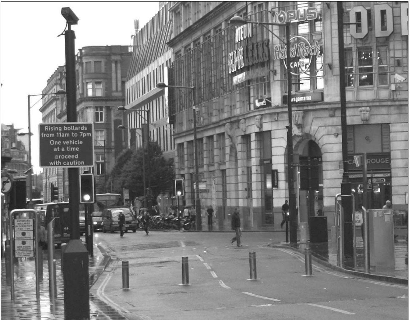
Fig. 1. A system of retractable bollards, which encircle Manchester city centre and limit access to vehicular traffic
