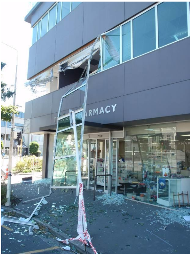
Figure 12: Disconnection of a light-medium weight cladding.
