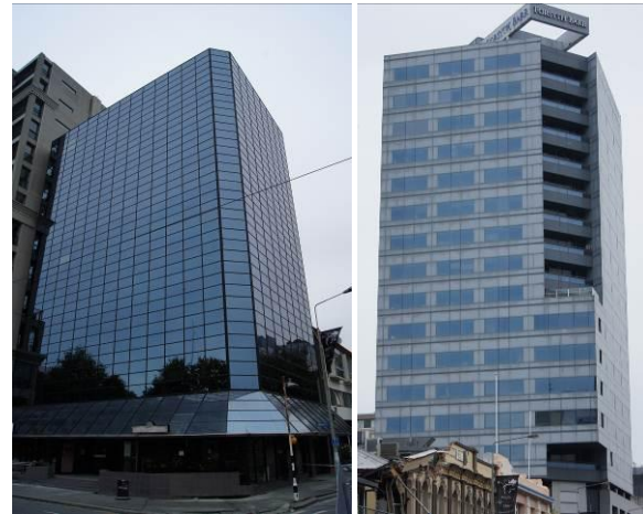
Figure 4: Examples of light-medium weight cladding present on Christchurch buildings.
