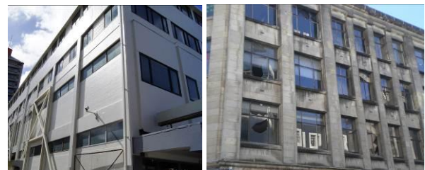
Figure 5: Examples of infill on Christchurch buildings.
