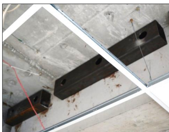
(b) Steel RHS at hollowcore floor unit support
