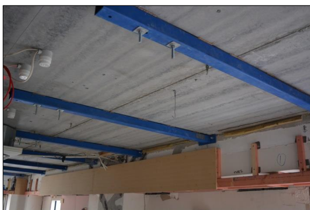
(c) Steel beams below alpha hollowcore unit
