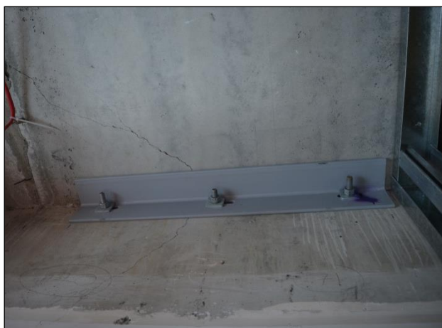
(a) Steel angle at hollowcore floor unit support
