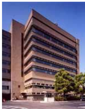
Photo 4 Building external view
