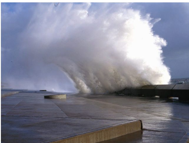
Overtopping of the seawall at Samphire Hoe (picture courtesy of the WhiteCliffs Country Project, taken October 1996)
