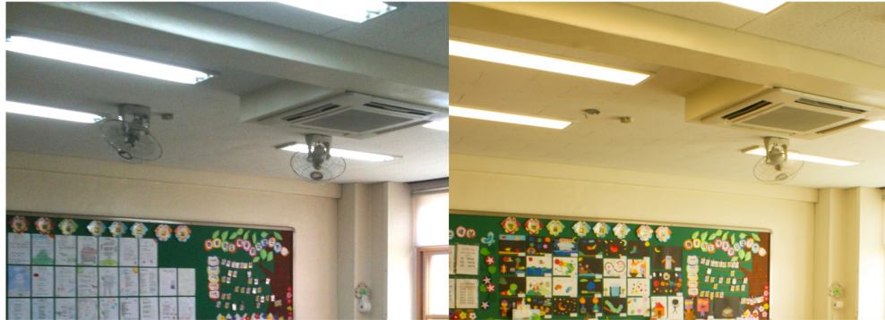
Fig. 4. The original fluorescent lighting (left) replaced with tunable LEDs (right).
