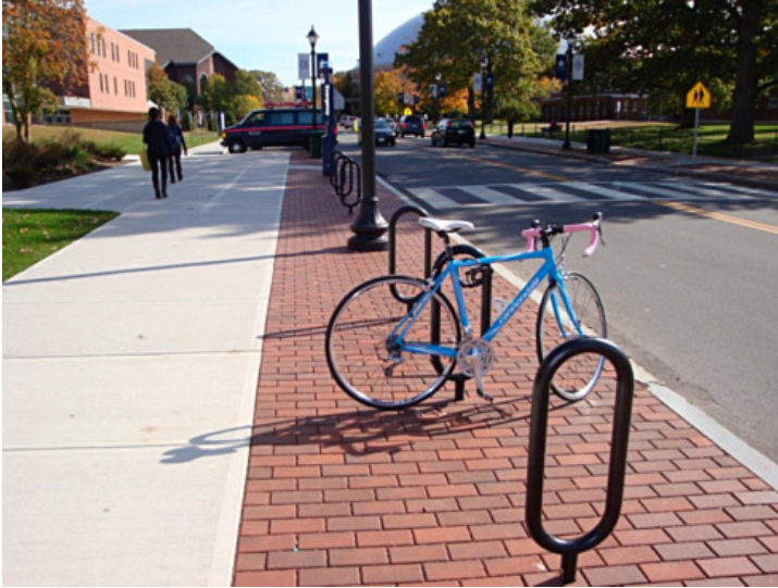
FIGURE 4: Pervious pavement in the “snow shelf” between the sidewalk and street, University of Connecticut, Storrs.
