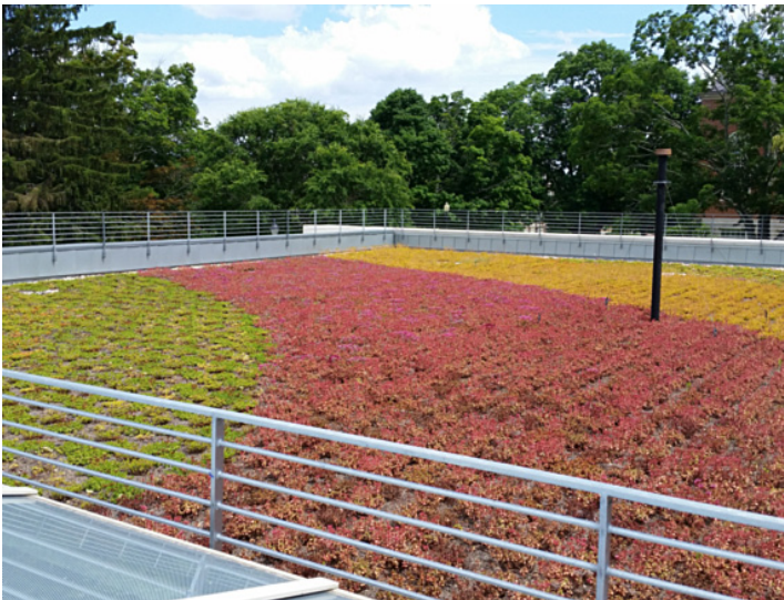
FIGURE 6: Green roof on Storrs Hall, University of Connecticut, Storrs.
