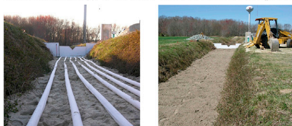
Fig. 1. Examples of different P sorbing technologies for addressing nonpoint P sources from agriculture, including (a) a preventive strategy whereby flue gas desulfurization (FGD) gypsum is applied to high P soils to immobilize water-soluble P and prevent P loss in surface runoff (photo credit: Ray Bryant); (b) two remedial strategies to remove dissolved P from soil water and shallow groundwater flow paths using a permeable reactive barrier filled with iron-coated sand (left) and enveloping a tile drain with iron-coated sand (middle and right) (photo credits: Wim Chardon and Gerwin Koopmans; see Chardon et al., 2012); and (c) a remedial strategy to remove dissolved P from concentrated surface flows in an agricultural drainage ditch using a FGD gypsum filter (photo credits: Ray Bryant; see Bryant et al., 2012).
