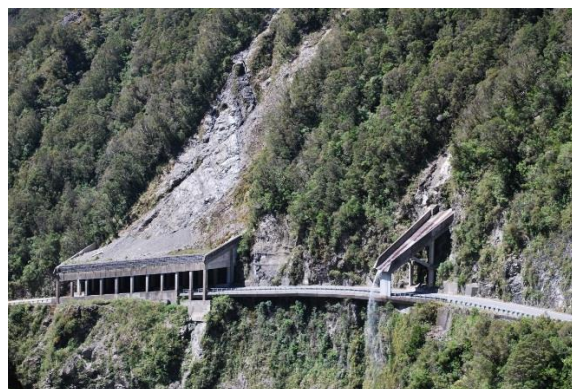
Figure 10: Otira rock fall shelter and aqueduct [34].
