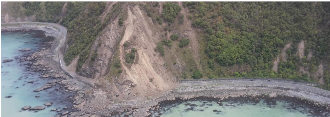
(c) Landslide on SH1, north of Kaikōura. Photo credit: Tonkin & Taylor
