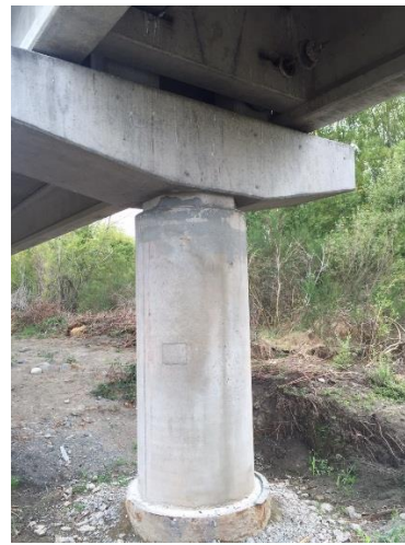
(d) Lower Mason bridge support repair. Photo credit: Liam Wotherspoon, UoA
