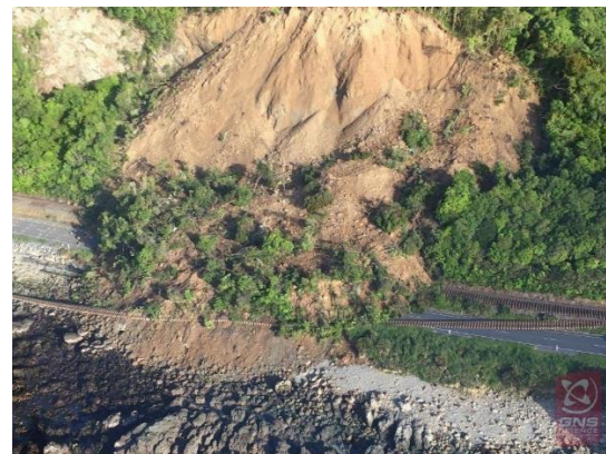
(d) Large offset of rail track due to landslide Photo credit: William Ries, GNS Science
