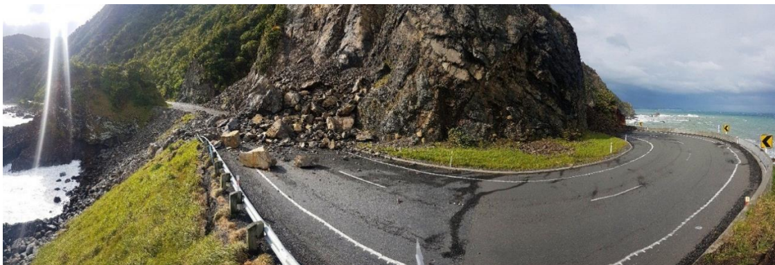
(d) Rockfall on SH1, north of Kaikōura. Photo credit: Dizhur & Giaretton
