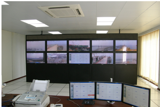
Figure 1: Construction project Video monitoring system.
