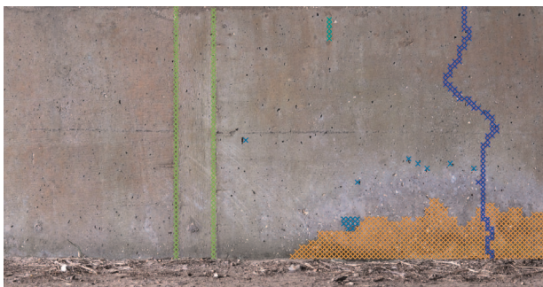
Figure 5. Example of a defect map overlaid on image, showing location and type of defect
